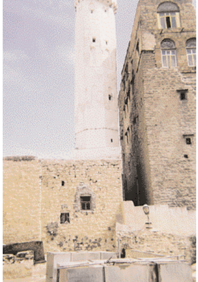
The Lrage mosque in the old Ibb.
