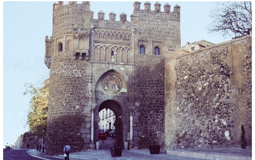
Another view of Bab As-Shams (Puerte del Sol)
