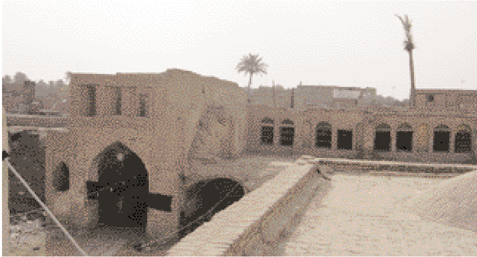
A view from the roof of the shrine
