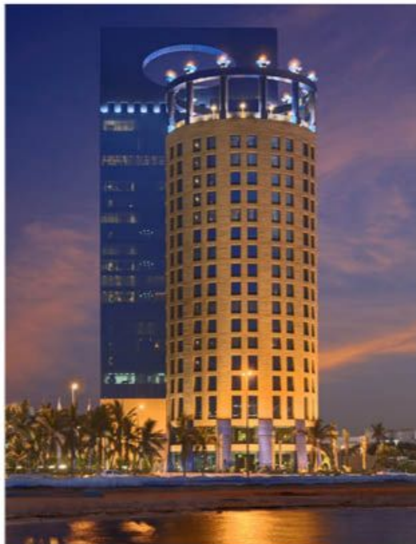
Rosewood Corniche - night view
